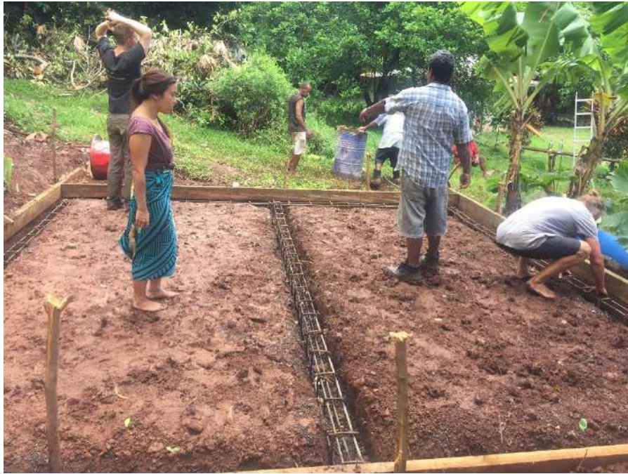
Figure 9 Thickened Sections
