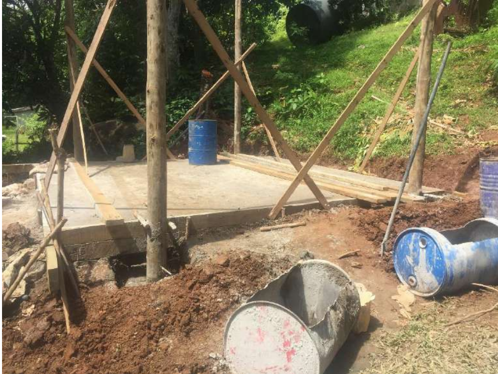
Figure 12 Installation of Posts
