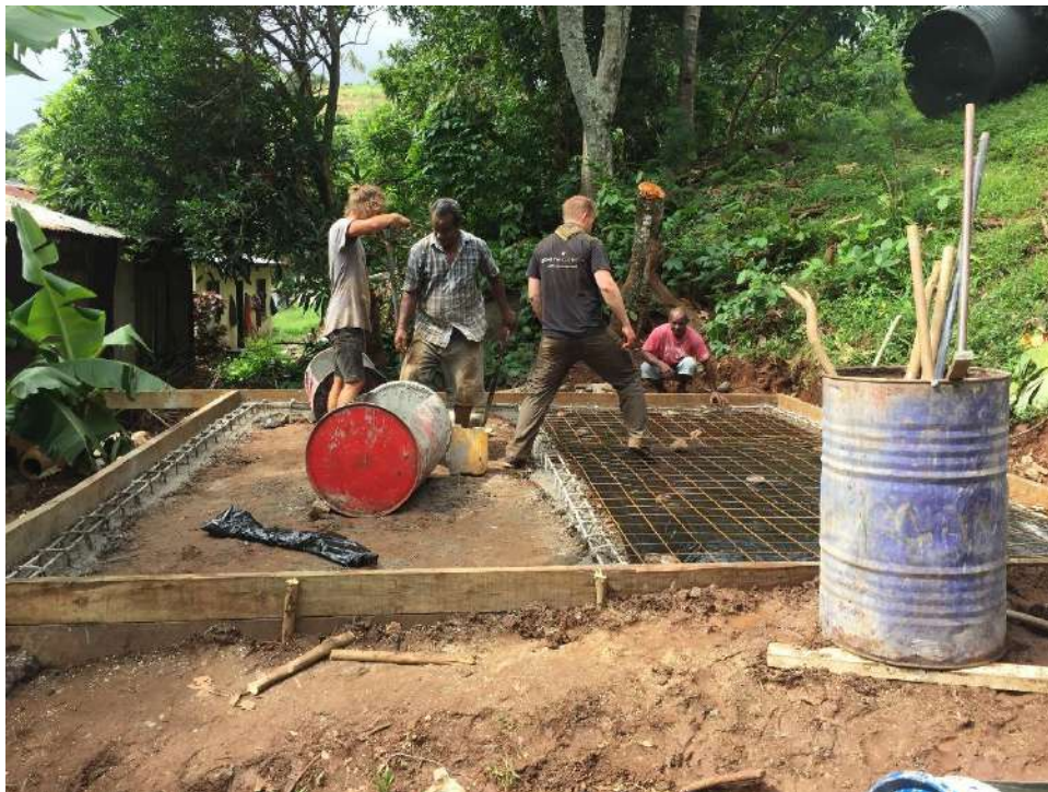
Figure 11 Installation of Plastic Membrane and Mesh Wire
