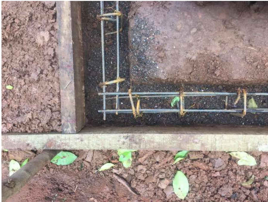
Figure 7 Rebar Placed on Compacted Gravel
