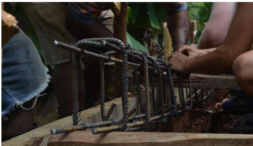
Figure 8 Rebar Stirrups
