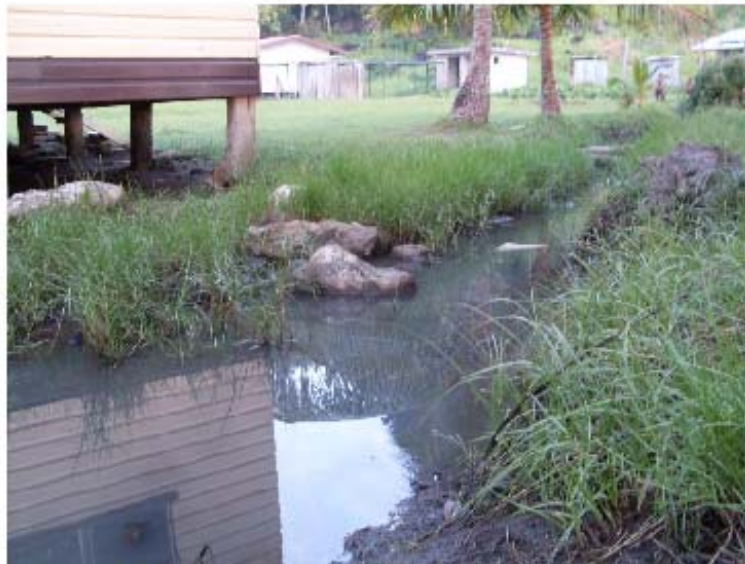
Figure 17: Open grey water trench in Ketei Village.
