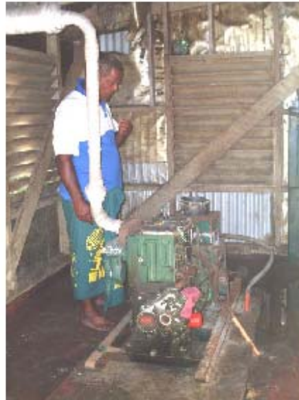
Figure 35: Diesel generator in Dravuwalu.
